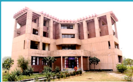
Central Institute of Nursing & Research centre Accommodation Block TNAI Headquarters
